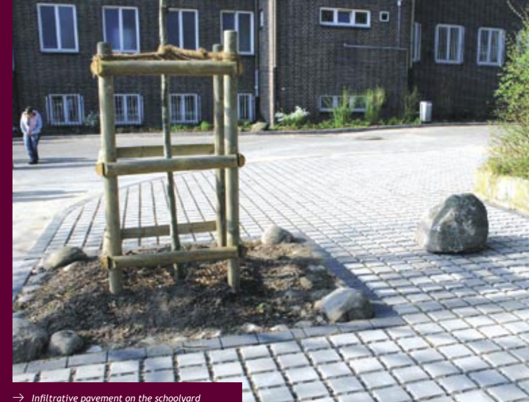
→ Infiltrative pavement on the schoolyard
